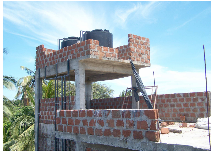
A new floor on Pastor Muralee's house
